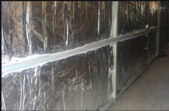
Wall framework and insulation.
