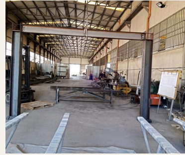
03 · Structure in progress.
