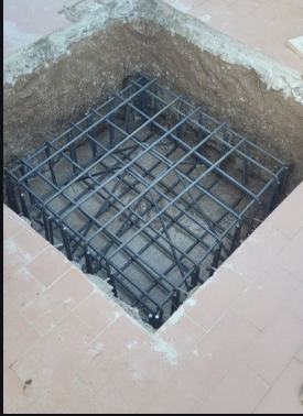
1 · Excavation and preparation.
