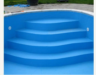
Completed stair detail.
