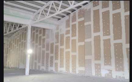
Interior works, systems and finishes in a retail environment.
