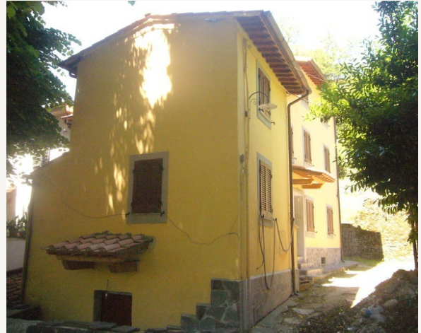
AFTER · refurbished and completed building.
