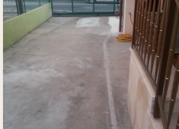
External paving • before.
