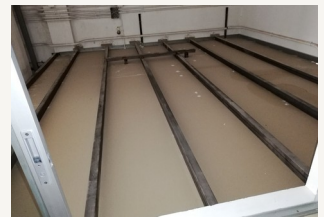
Suspended-ceiling framework and metalwork.
