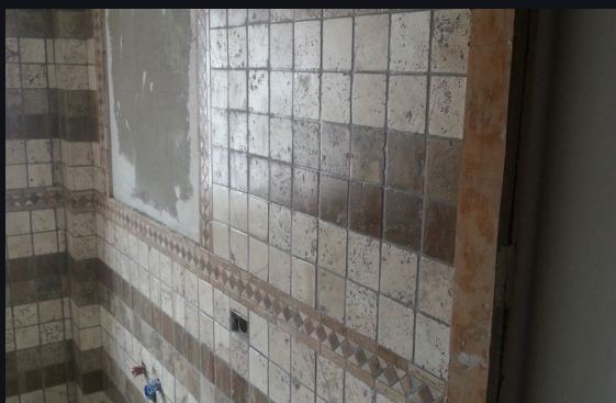
Colleferro bathroom · before.
