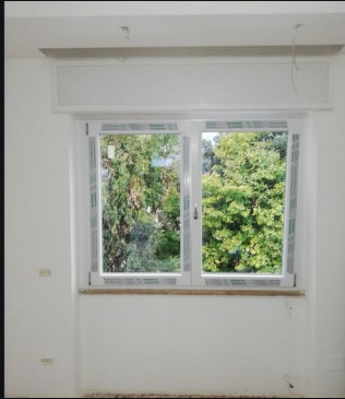
Window/door system + drywall · integrated works.
