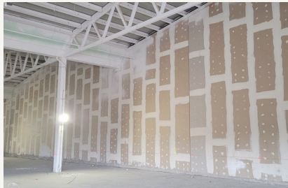
Coordination of construction and technical systems in complex commercial environments.
