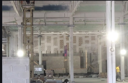
Large retail space during construction and coordination.
