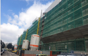
Façade • metalwork and painting.
