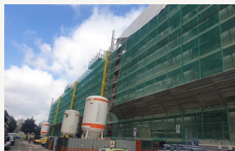
Façades, metalwork and painting.
