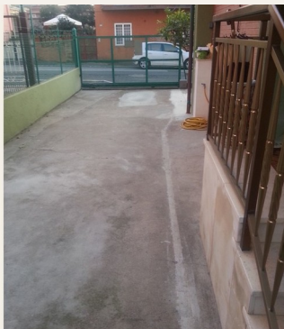
External paving • before.
