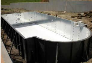
Pool during construction.
