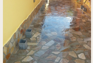
External paving • after.
